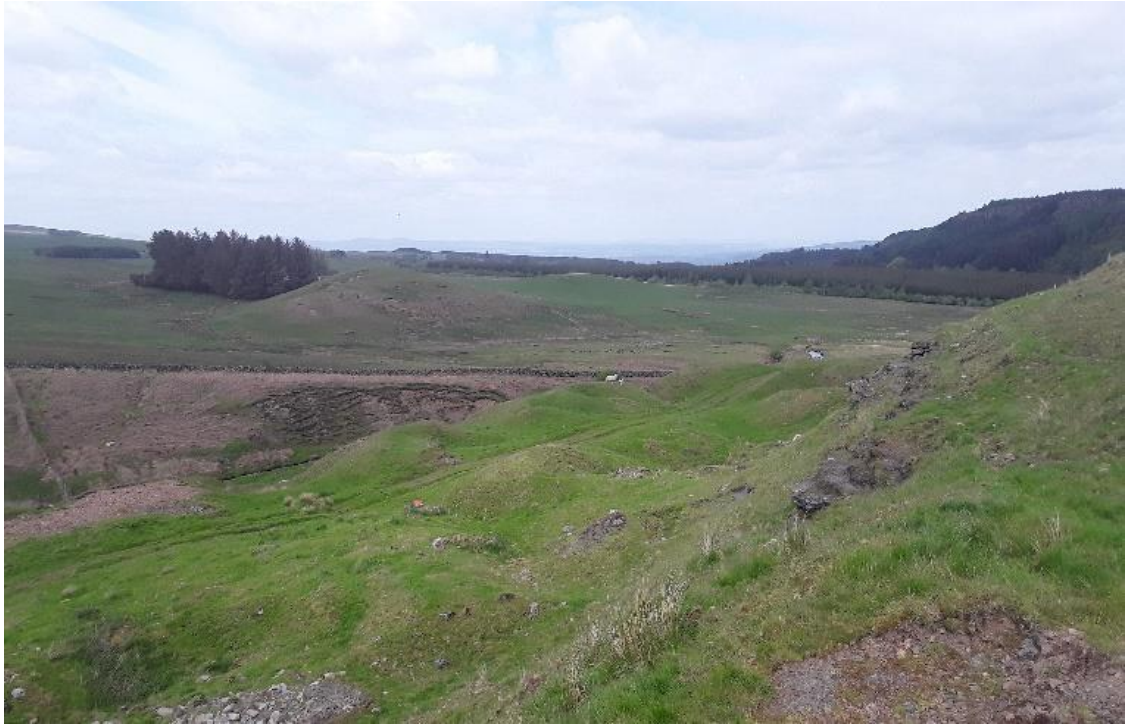
Plate 10A-8: View looking northeast of the quarry faces and clamp kiln to the south of the Bannock Burn
