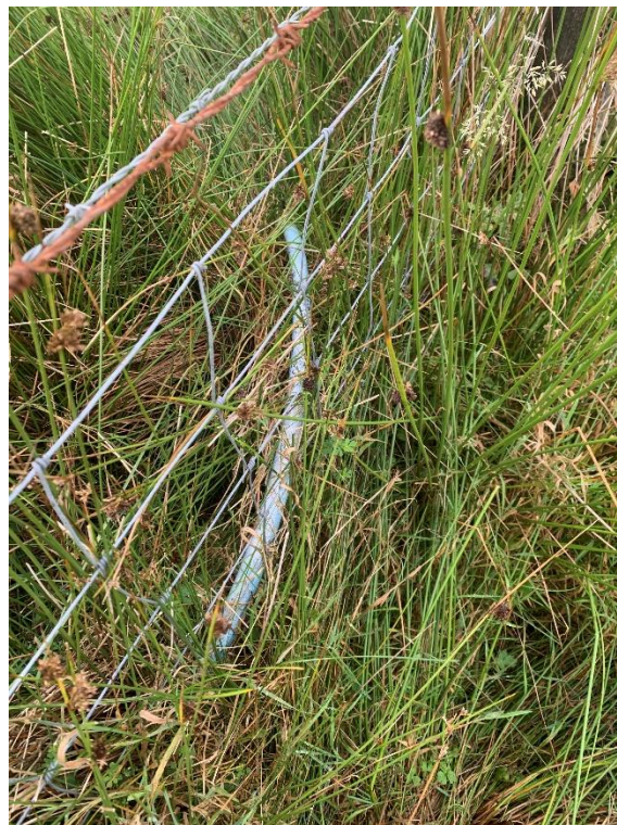
Figure 3: Exposed pipework where it crosses a watercourse, between header tank and supply.
