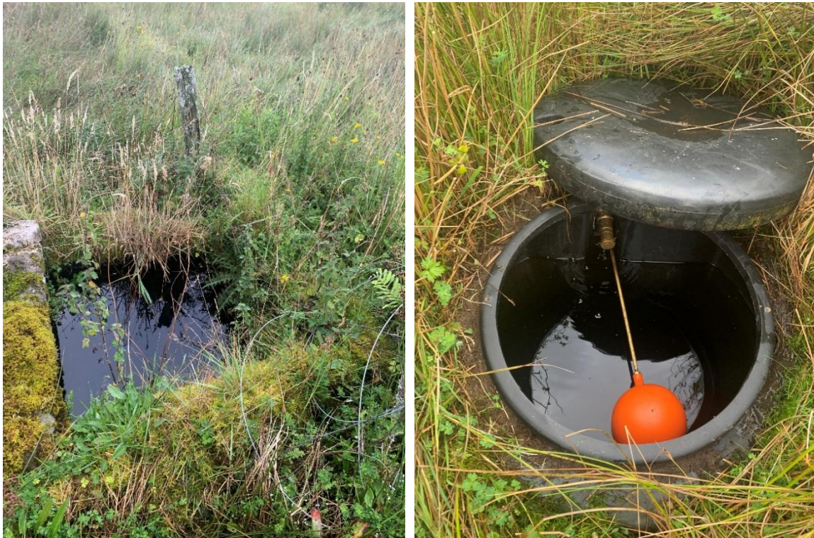
Figure 1 and Figure 2: PWS source tank (left) enclosed by brick and, left open. It is connected to the header tank by pipe. The header tank (right), which is covered and has a ballcock valve. The water is then piped to downslope to the supply at the property.
