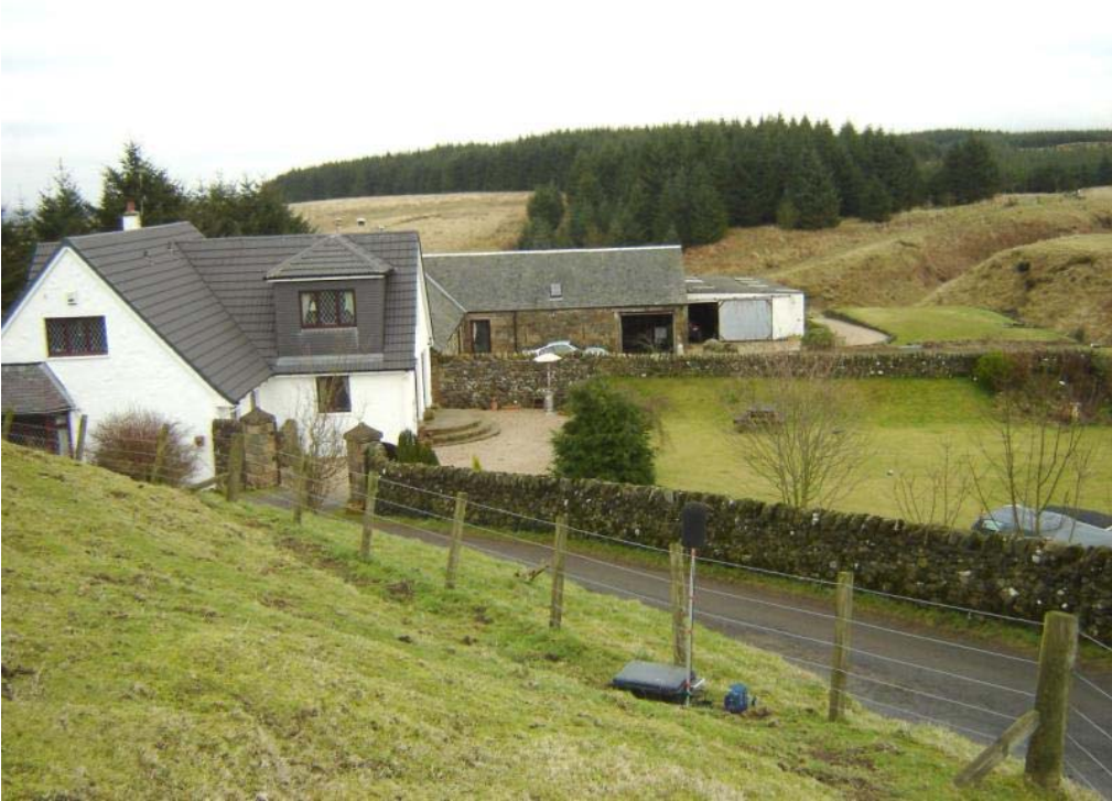
Figure A2.31 View of the monitoring location at Carrot looking East.
